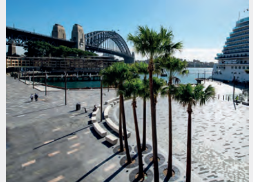
The Campbells Cove Redevelopment at The Rocks in Sydney, planned and designed by SJA.
